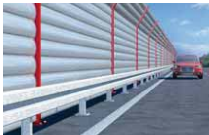
Crash barriers and sound insulation walls
