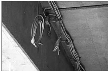
X-ECH for fastening bunched cables
