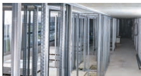
Drywall tracks to concrete and steel
